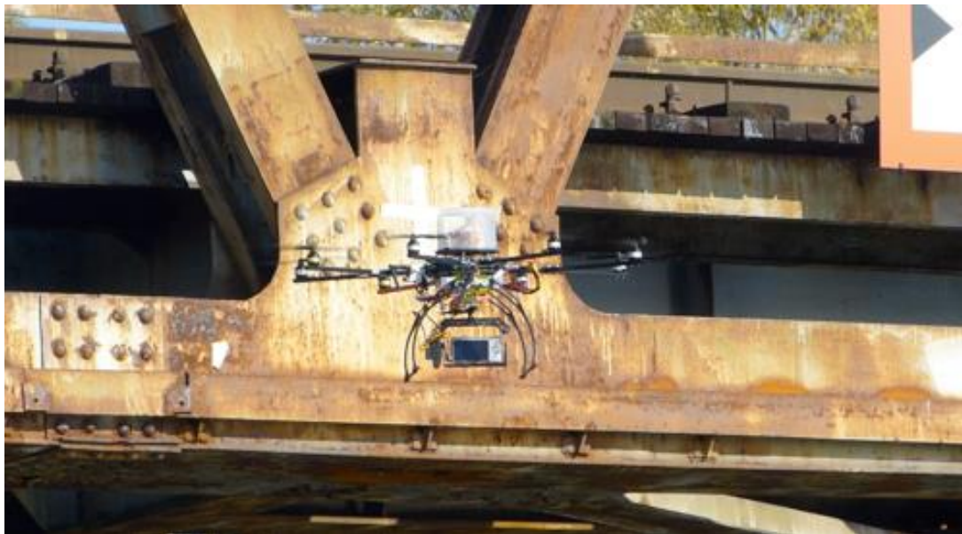
Fig. 3. Infrastructure inspection using our developed UAV equipped with a camera.
