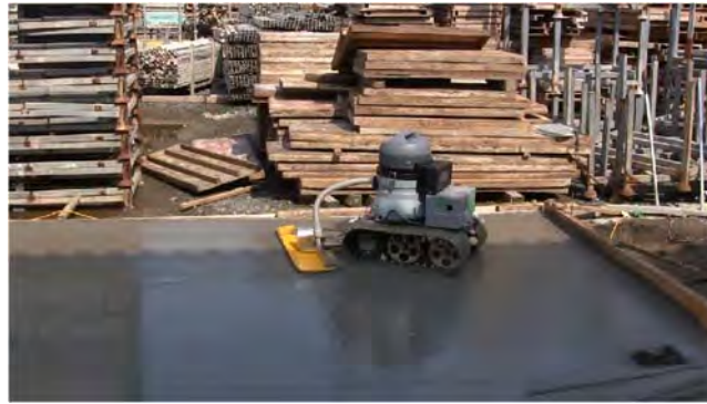
Figure 1. Mobile robot working on a concrete surface
